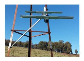
6) Attach a bracing arm from the main rail (M12 bolt) across to the most suitable position. (Ends may be bent/twisted to align as needed).
